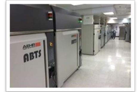
Packaged Part Test & Burn-in Production
